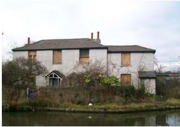
Front elevation from the Canal
