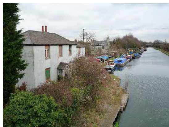
Front elevation from Bull's Bridge
